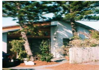
Residence, Lennox Lane, Lennox Head
