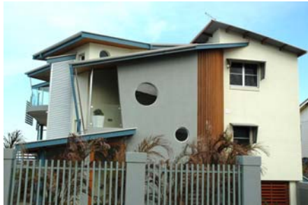
Sanbah Apartments, Rayner Lane Lennox Head
